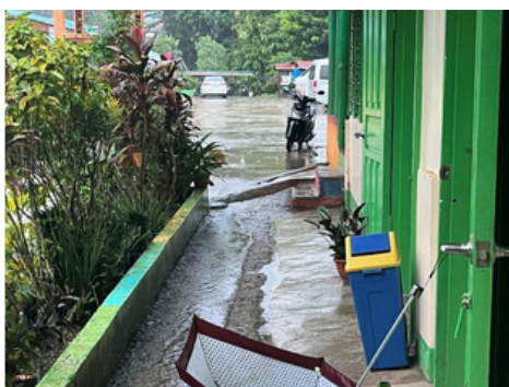
Figure 3. Condition of the elementary school, recorded at 15:08 (PST), showing side gutters in front of the classrooms nearly overflowing after 44.6 mm of rainfall within 30 minutes.
