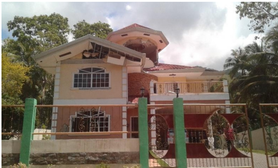
Figure 2. A few meters from the Segundo House, this RC-framed masonry house visibly incurred significant damage after the earthquake.
