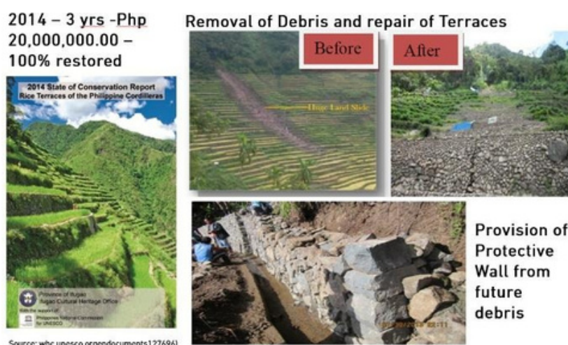
Figure 2. 20 Million Pesos was the amount of the repairs for the 2011 landslide. The debris was removed. Terraces were rebuilt and the wall between the Muyong and the terraces were repaired for the purpose of protecting the terraces from future debris if it ever erodes again.
